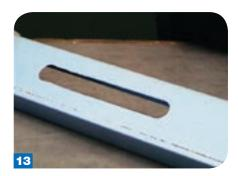
The finished penetration slot, in this example, made by an electric nibbler.
