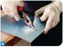
When cutting, don't take large bites. Cut with small cuts (approximately 5–10mm) moving the blades forward to create a neat and continuous cut.
