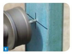
To drill a penetration hole in a **boxed stud** first locate the centre point for the hole on one side of the stud and drill.
