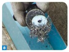
Hole cutting creates swarf. Remove swarf to avoid risk of corrosion. For a professional result, clean up any swarf on the surface of the metal. Use a magnet to efficiently remove swarf from the base plate.
