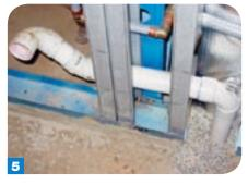
Drilling back-to-back C-channels is simple.
