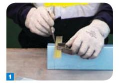
Notching noggins. If you need to notch out a noggin, use a ruler or template to mark out the line to be cut. We recommend you use tin snips to cut out a noggin. See Hand cutting light gauge steel with tin snips.
