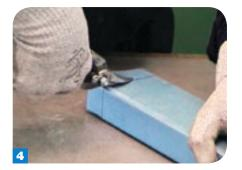
With the same snips, cut along the line to the opposite corner. Then use the right cut snips to cut into that corner.
