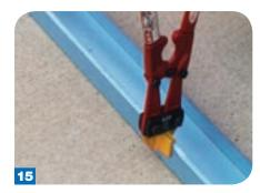
It is a simple tool that is used to flatten the lip as opposed to cutting it out, saving time on the job.
