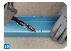
Then use both left and right snips to cut out the material on both lips.
