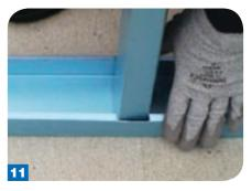
**Notching lip C-channel plates.** Notching lip C-channel plates to insert a stud can be done easily by using left and right cut snips.
